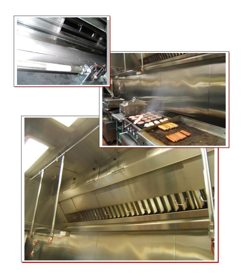
THE UVC SYSTEM IS DESIGNED TO BE USED WITH CADDY'S NEW HIGH VELOCITY MULTI CHAMBER CARTRIDGES. DEPENDING ON THE EXHAUST REQUIREMENTS THE INTAKE SLOTS CAN BE POSITIONED AT THE TOP OR BOTTOM OF THE HOOD INTERIOR. STAINLESS HANDLES PROVIDE EASY REMOVAL.
