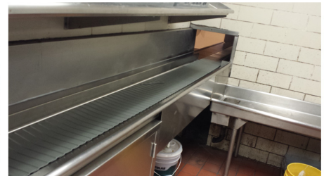
COMPLETED BELT TO DROP-OFF
