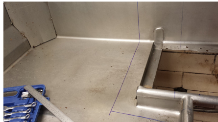
CUTTING OUT DISH TABLE
